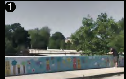
Randolph St Bridge
